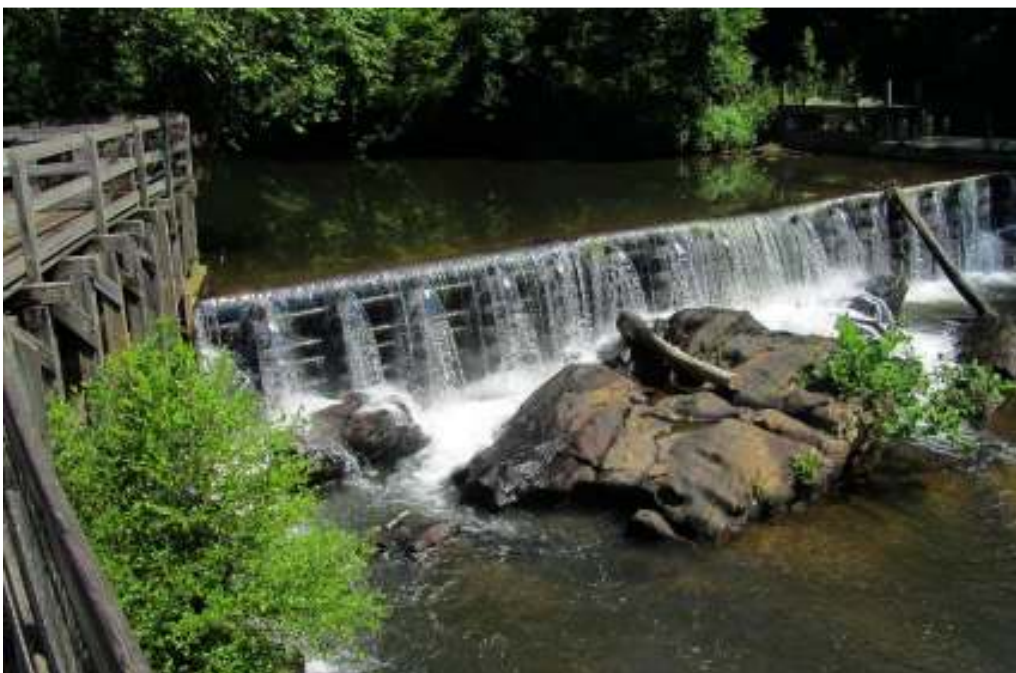
Nora Mill Dam on Chattahoochee
